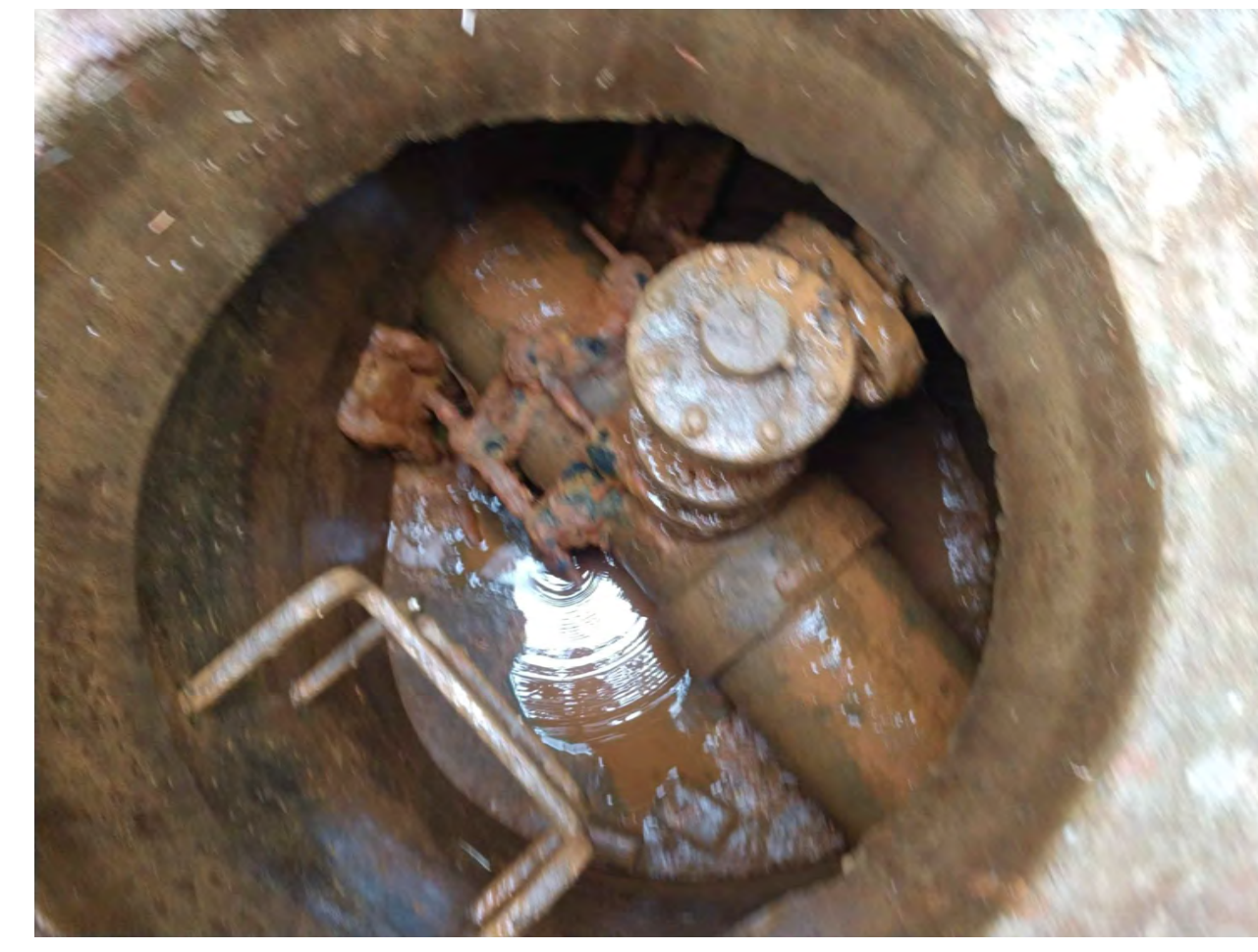
ACCESS POINT-1 INSPECTION PHOTO
