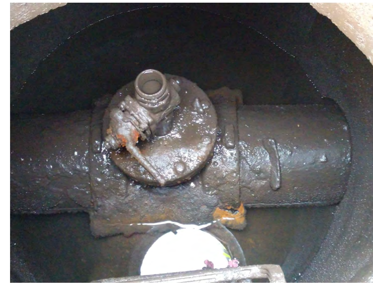
ACCESS POINT-3 INSPECTION PHOTO
