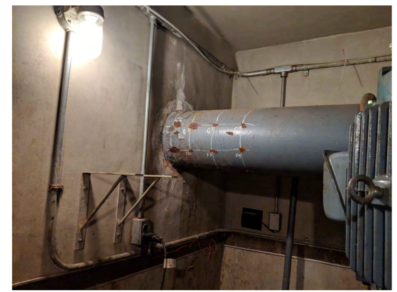
PUMP STATION INTERIOR - EXISTING FORCE MAIN OUTLET
