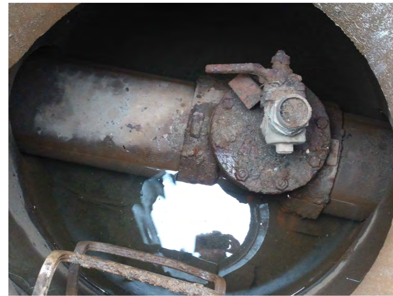
ACCESS POINT-2 INSPECTION PHOTO
